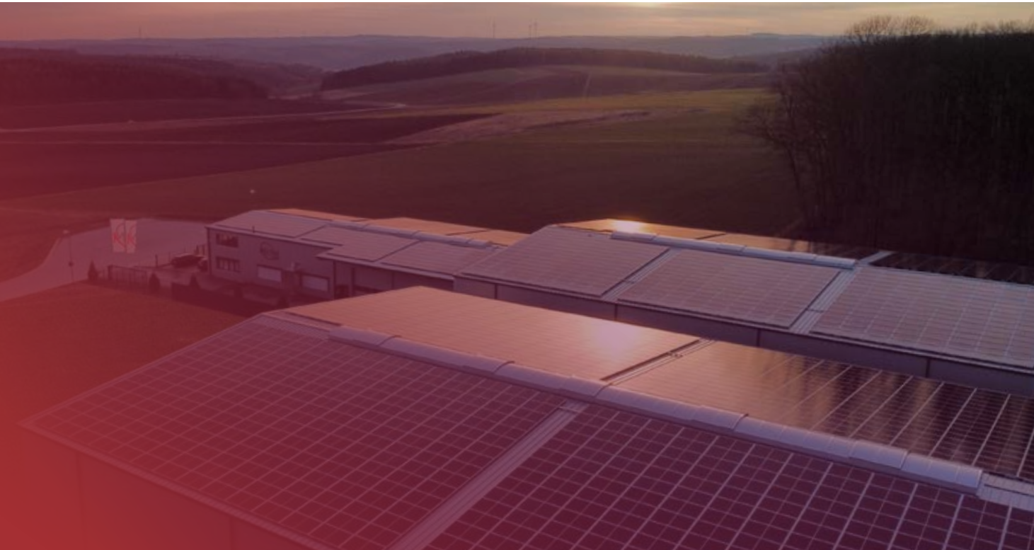
Headquarters of Michel Tube Engineering GmbH in the A81 industrial park
